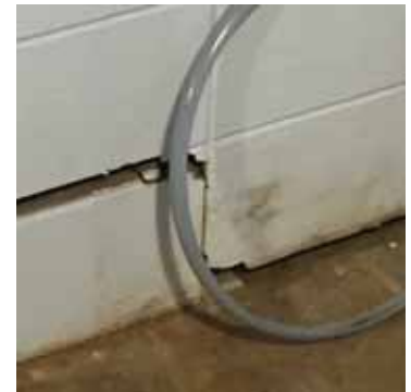
Block Wall Failure
